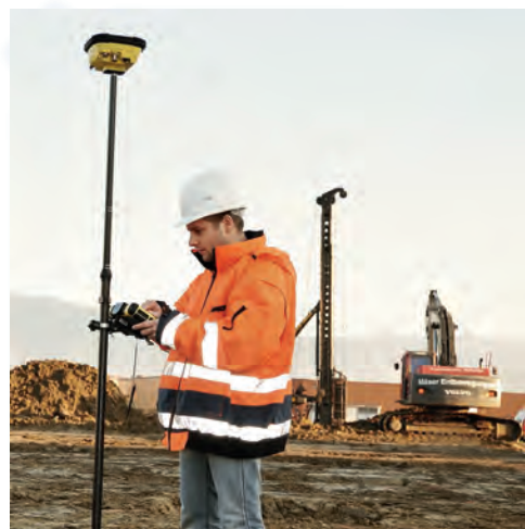
Survey and Construction Positioning with RTK Corrections
